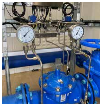
The left image shows the AVK Series 879 diaphragm control valve fitted with VIDİ flow and pressure sensors.
